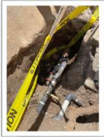
New water shut-off valves
